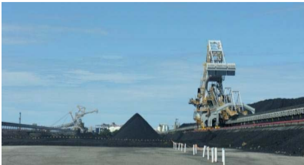
Coal Stockyard: Stacking and reclaiming facilities
