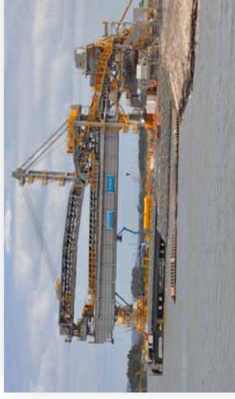
Train Load-out system under construction
