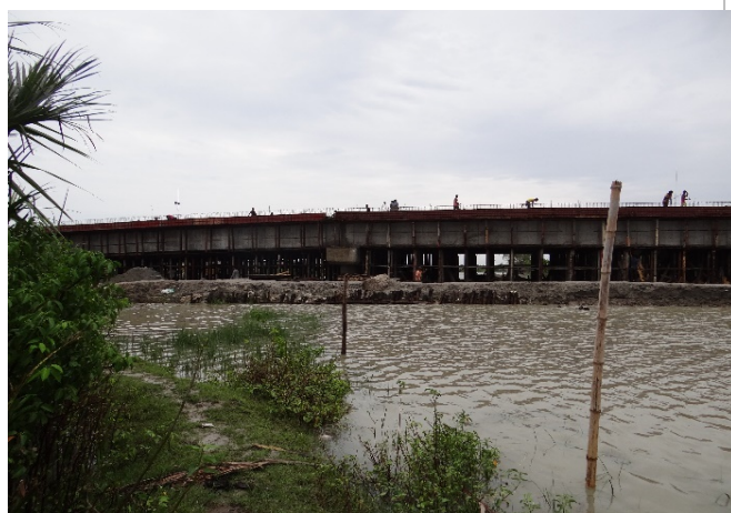
Temporary cross-dam over Maidara River restricting natural flow
