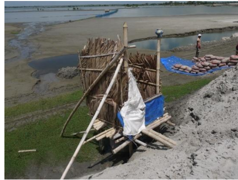
Open Pit Toilet installed at construction site, contaminating nearby water bodies
