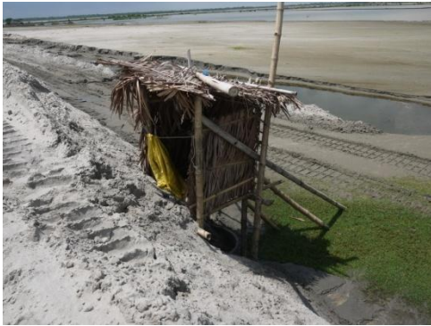
Open Pit Toilet installed at construction site, contaminating nearby water bodies
