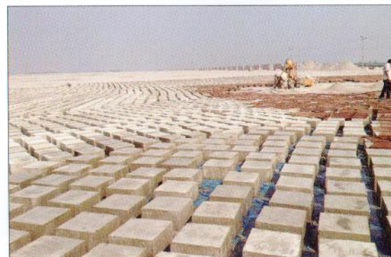
25 November 2014 Cement Concrete Block for Slope Protection Work in progress at Site
