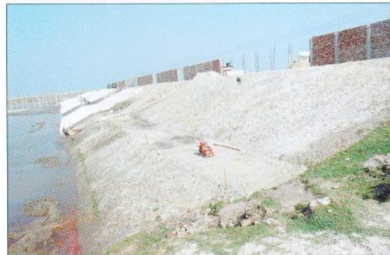
04 November 2014 Slope Protection beyond Boundary Wall in progress
