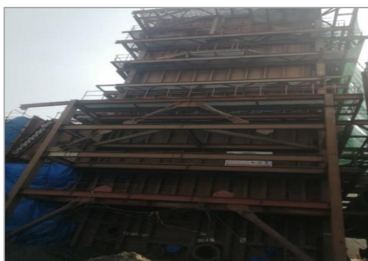
Construction of FGD
