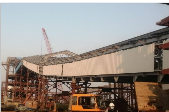
Construction of closed coal conveyor belt
