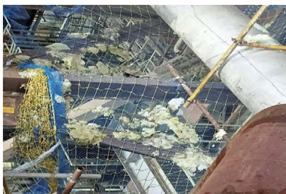
Figure 4.1: Unsafe asbestos management
