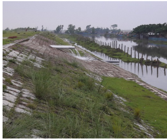
Figure 3.2b: Storm Discharge Water Outlet
