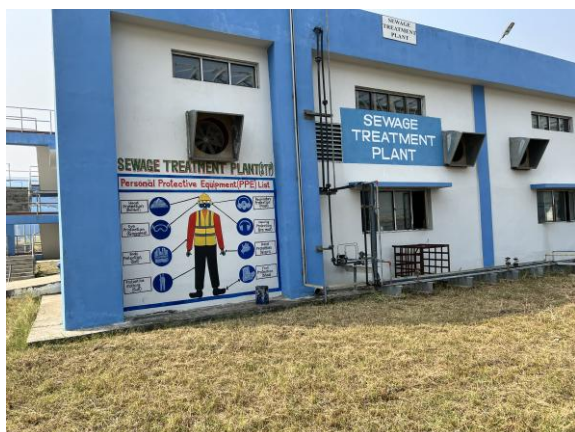
Sewage Treatment Plant
