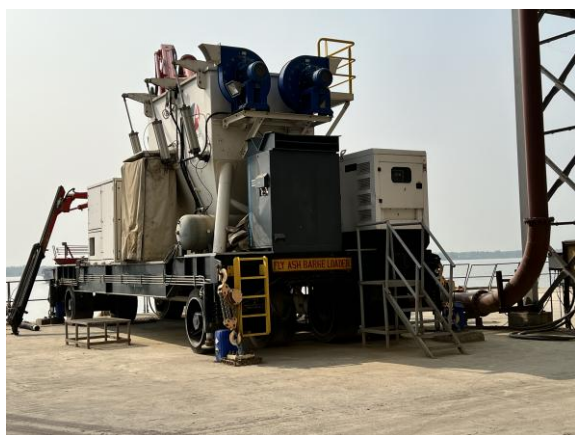
Fly Ash Barge Loader
