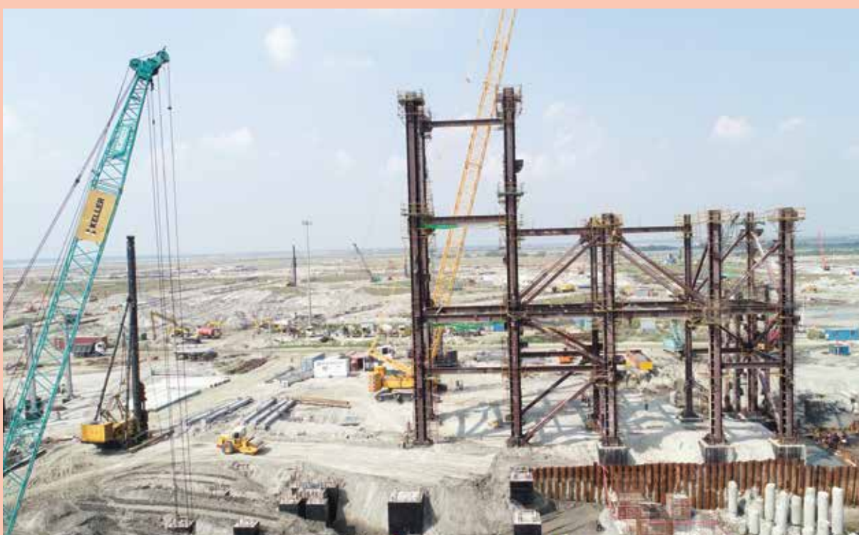
Boiler Erection (Unit # 1)
