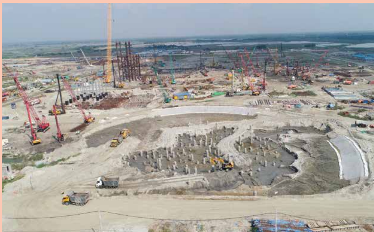
Chimney Pile Excavation
