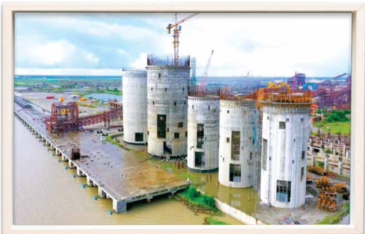
Gypsum, Bottom Ash & Fly Ash Silo
