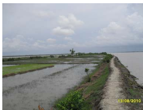
Plate: Earthen Levee along the Passur river to prevent tidal intrusion in the Project area
