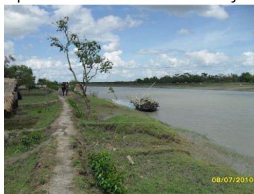
Plate: Earthen Levee along the Maidara river to prevent tidal intrusion in the Project area
