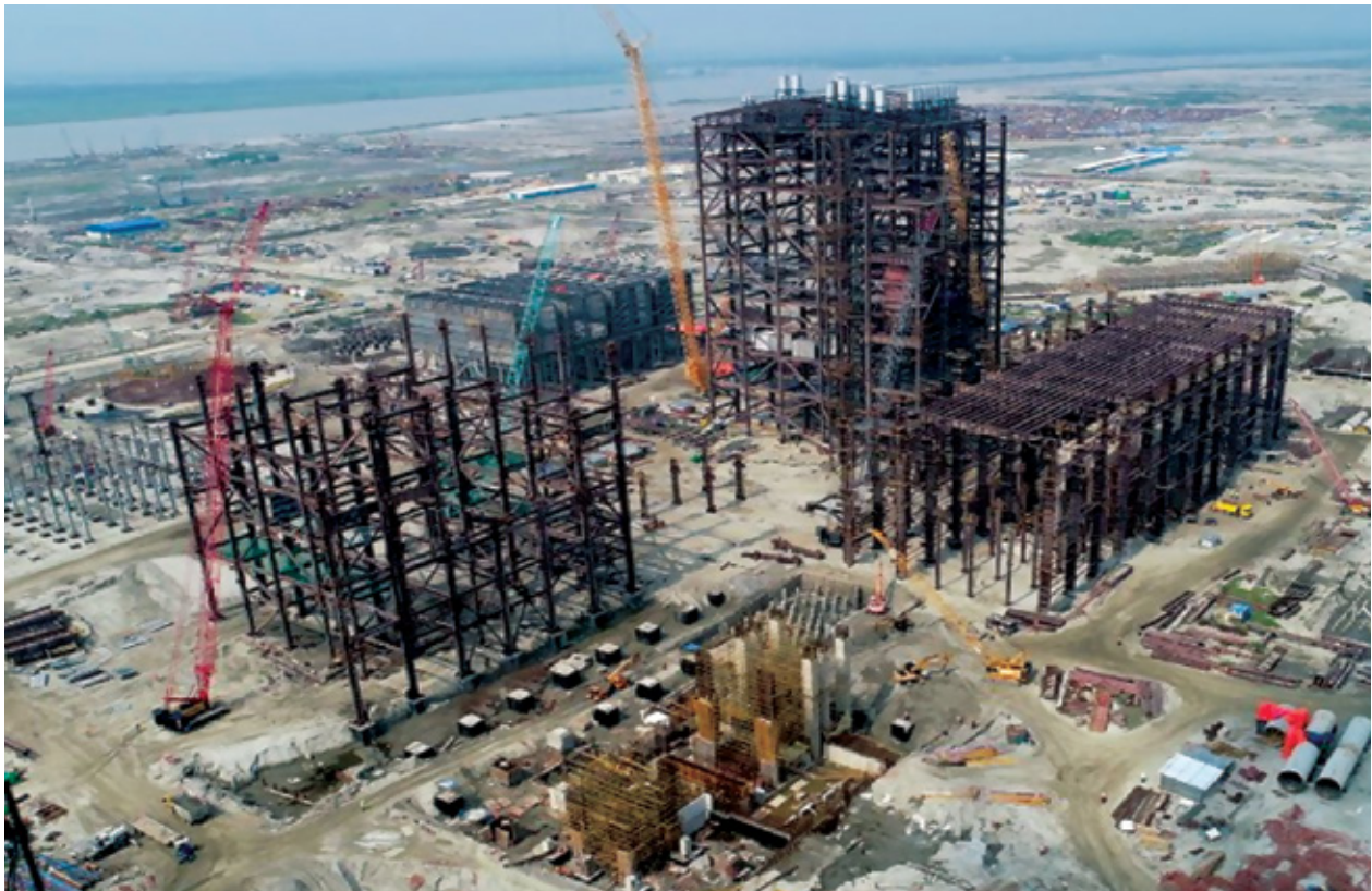
Erection of Boiler (Unit # 1 & 2)
