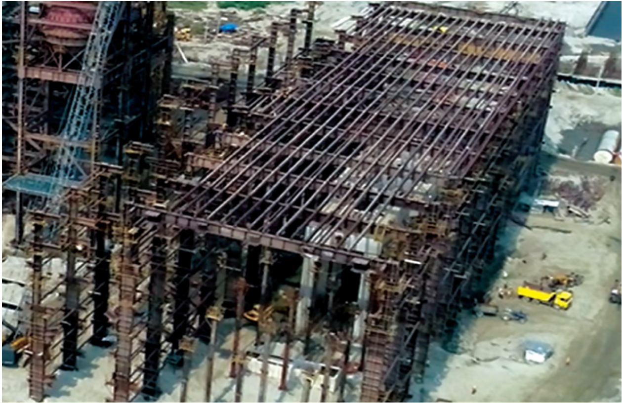
Erection of Main Power House (MPH)
